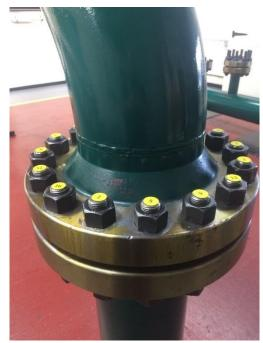
The TorqTag is scanned with the COMMANDER prior to torqueing to ensure the wrench is on the correct bolt.
